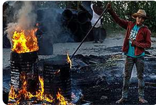
Strassenbau in Mawlamyine
