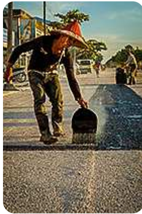
Strassenbau in Mawlamyine
